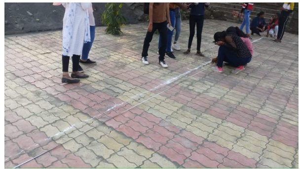
Layout of Foundation of Residential Building of Construction Technology Practical on 28th October 2021
